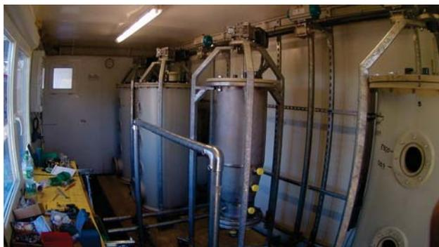
Figure: Container 2 with hydrolysis reactor and fermenters
