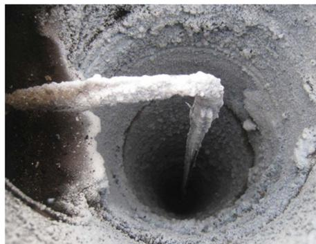
Figure 1: Deposits of particulate matter around ESP in a chimney
